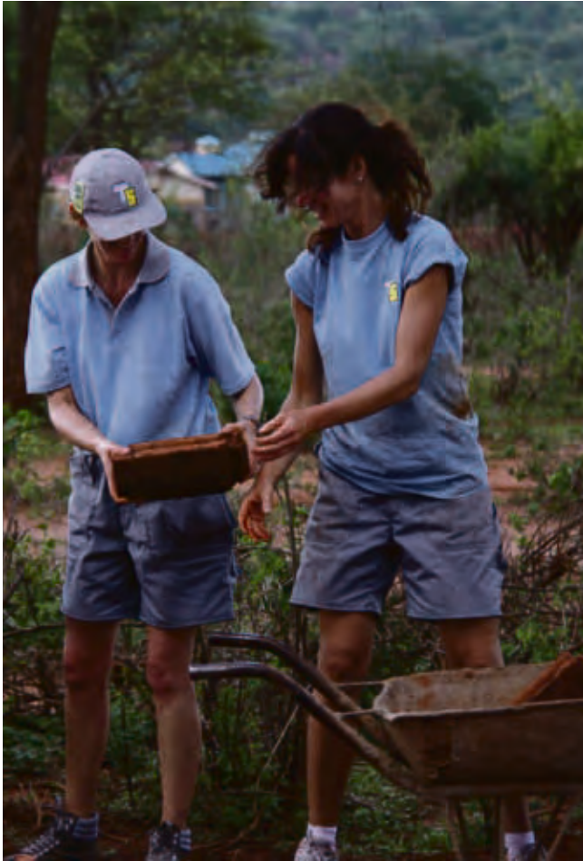
'Ter Steege' construction workers assisted in a Housing project in Wikivuvwa, Kenya.
